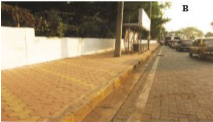
9.3 Area with garbage vs clean area
